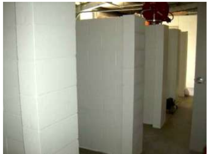
Midcoast shelter—dog runs being built
